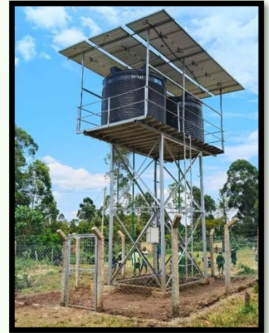
A water tower similar to the one planned for Children of the King
