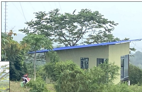
Mountain radio station exterior view
