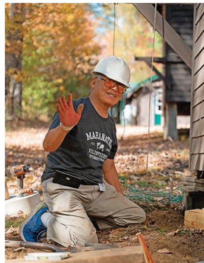
A volunteer reinforces a cabin foundation.
